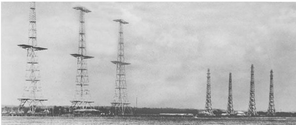
Chain Home stations consisted of four 360ft high metal transmitter towers and four 240ft high wooden receiver towers. Chain Home Low varied between 20ft and 185ft depending on geographical surroundings.
